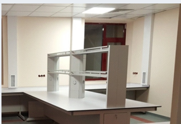
Absorption application directly from work area
